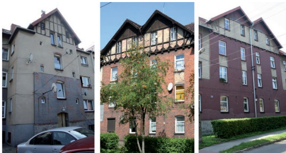
II.5-7. View of the residential buildings in the railway settlement in Pyskowice, an originally non-usable attic made of the Prussian wall, A. Szymanowska-Gwiżdż, 2014
