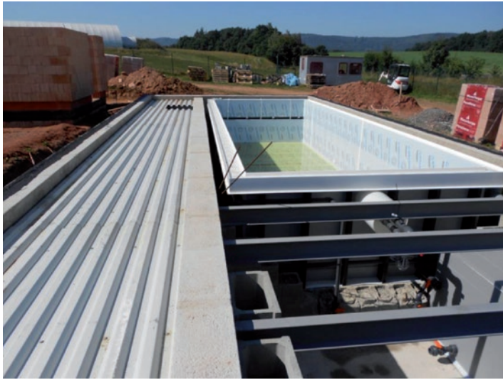
Figure. 7 Construction in August 2016. Photo: M. Nedvěď
