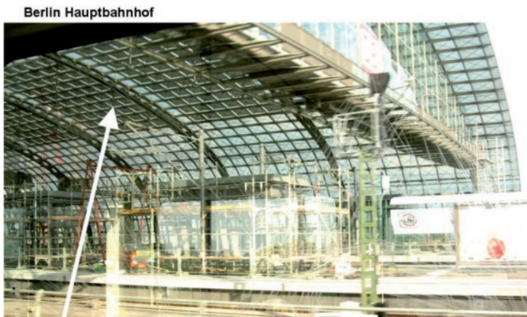
II.3. Photovoltaic components installed on the glass roof of the central railway station in Berlin. (photo Anna M. Włodarczyk, 2014)
