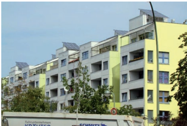
II.5. View of the photovoltaic panels installed on the roof of the buildings of High-Deck settlement in Berlin.
