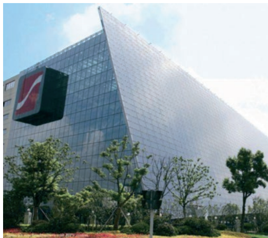
Il. 5 Research and Development Centre, Wuxi Suntech Power, Wuxi. BPV glass façade is created by 2552 semi-transparent photovoltaic panels with a total area of 20 000 m 2 . Photo Suntech [5]
