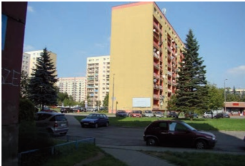
II.14. Peak wall of the building.
