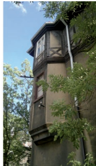
II.2-4. Wooden details of the Prussian wall in the residential buildings in Zandka settlement in Zabrze, A. Szymanowska-Gwiżdż, 2016
