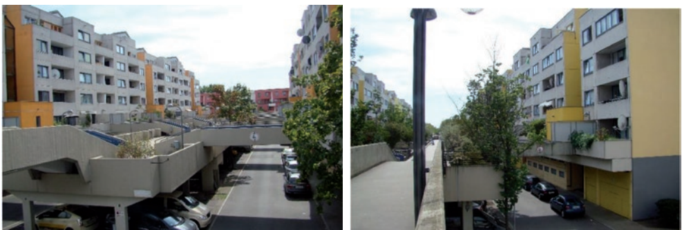
II. 1.; II. 2. Street view of High-Deck settlement in Berlin. Source: photo by Joanna Biedrońska August 2015.
