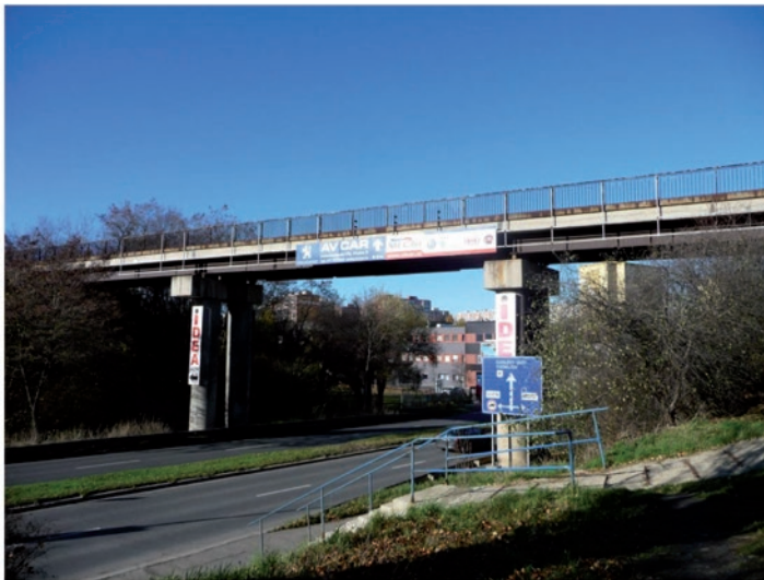
Figure 5: The side view of the railway bridge in Prague
