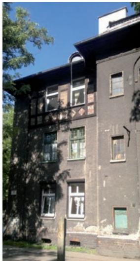
II.2-4. Wooden details of the Prussian wall in the residential buildings in Zandka settlement in Zabrze, A. Szymanowska-Gwiżdż, 2016
