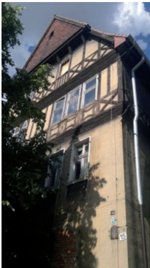
II.2-4. Wooden details of the Prussian wall in the residential buildings in Zandka settlement in Zabrze, A. Szymanowska-Gwiżdż, 2016
