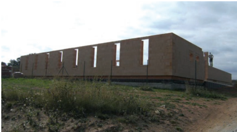
Figure. 8 Construction in September 2016. Photo: M. Nedvěď
