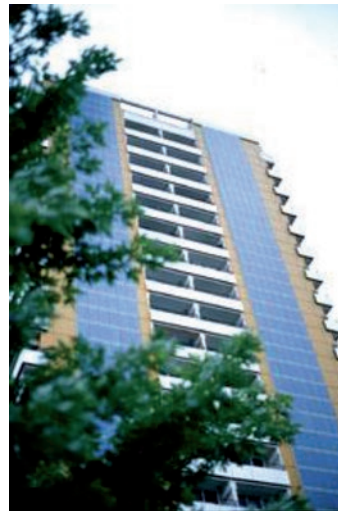
II.9. View of the façade. Source: [9].
