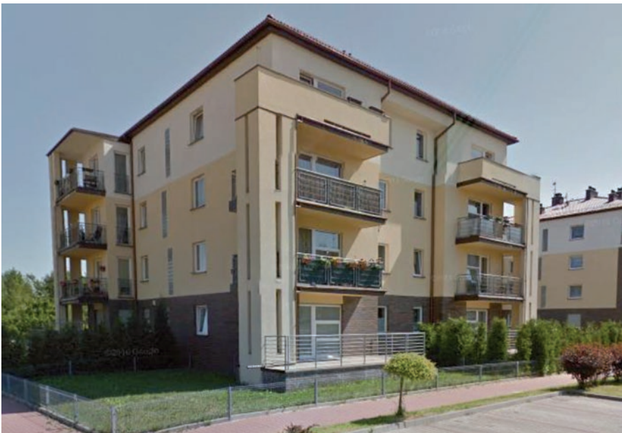
Photo 1. View of the façade of a typical building for which this article was developed.
