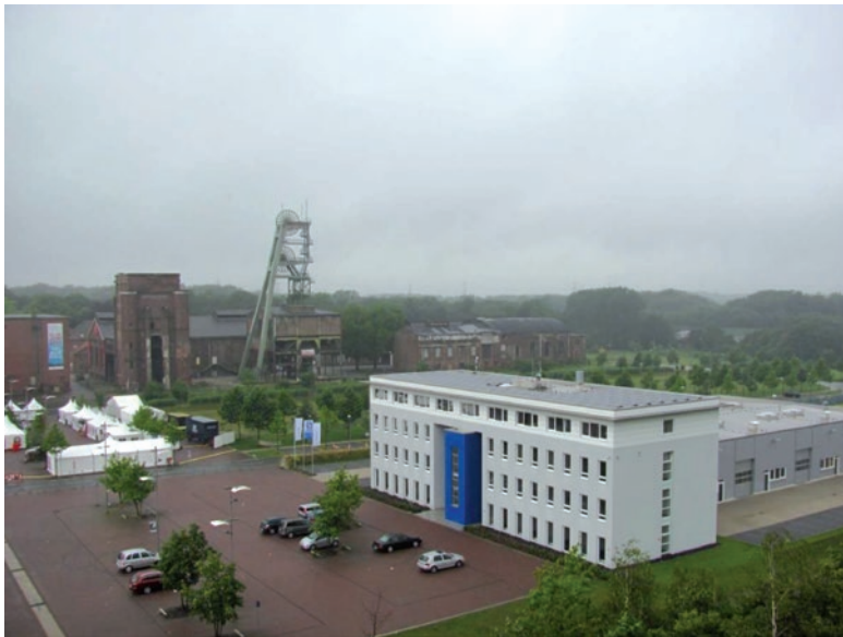
Figure.3 The new construction on site Ewald in the Herten - on the roof of the new object photovoltaic panels are placed, Vojvodikova, 2011
