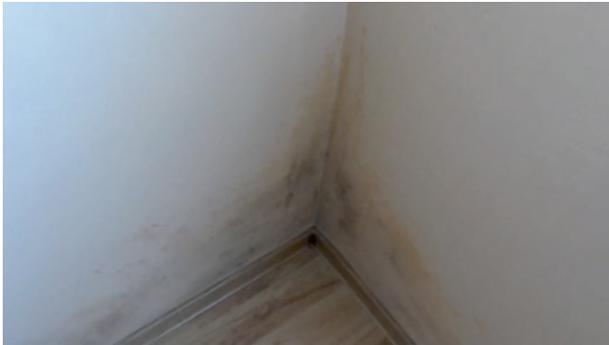
Il. 5. Dampness and mould in a corner of a room on the ground floor (the author).
