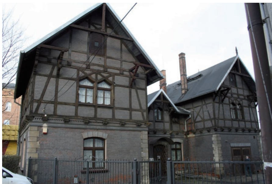
II.8. The Prussian wall in the building of the State Music School in Gliwice, A. Szymanowska-Gwiżdż 2015
